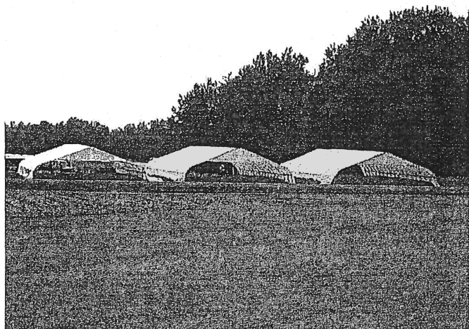
Figure 1. Three rain exclusion shelters at the Tidewater Agricultural Research and Extension Center in Suffolk, VA, accommodating peanut irrigation research.
